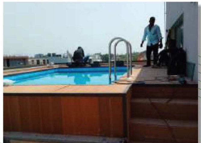
ROOF TOP DECK
