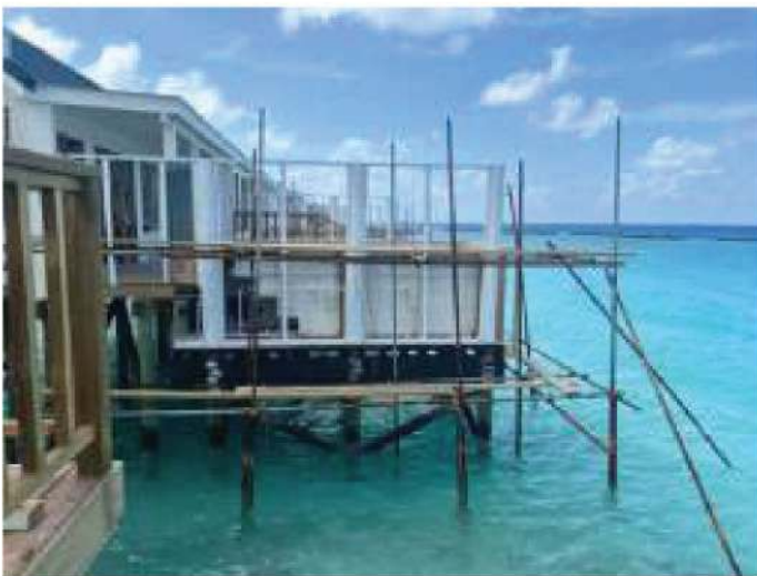
WATER VILLA POOLS, OPPO 36 POOLS MALDIVES
